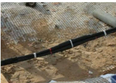
TS-24CSJ hybrid transition joint
