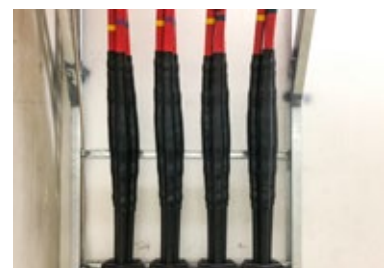
24CSJA-S cold-shrinkable straight joint
